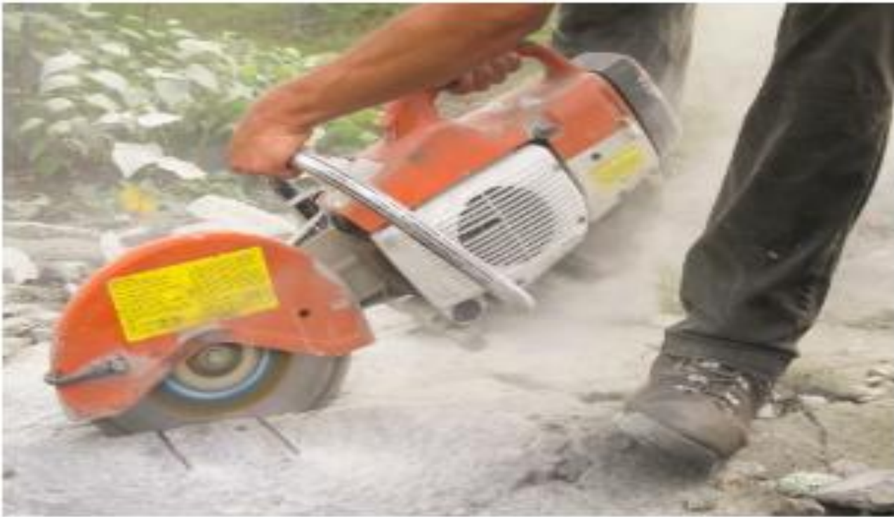
Figure 49: Groove Cutters and Edger's
