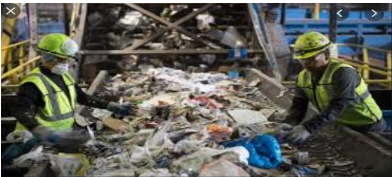
Figure 100: disposal of excavated material
