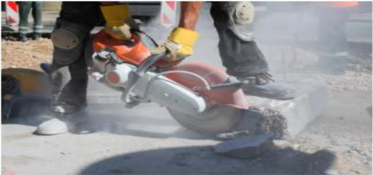
Figure 48: concrete saws
