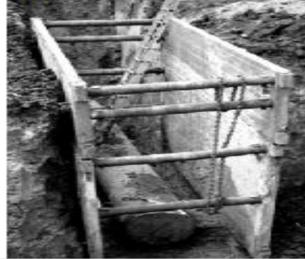
Figure 45: Shoring and shielding of cave in
